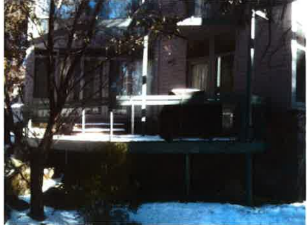
Figure 6: Photo of the north-east elevation and existing deck to be renovated
