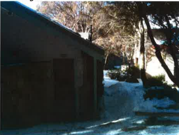
Figure 9: Photo of the rear south-west corner and location of proposed spa
